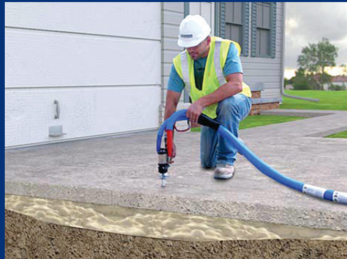
EXTERIOR SLAB LIFTING
