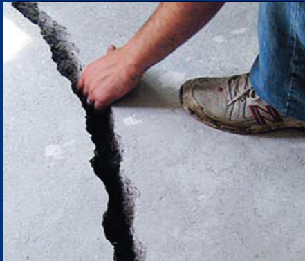
INTERIOR SLAB FLOOR LIFTING
